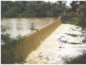
The weir at Coburg Lake in Victoria (Australia) after heavy rainfall.
