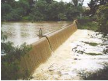
The weir at Coburg Lake in Victoria (Australia) after heavy rainfall.
